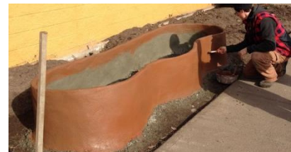
Figure 3: Curvy ferrocement beds
