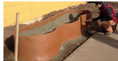
Figure 3: Curvy ferrocement beds
